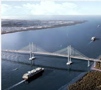
New Demerara River Bridge Georgetown, Guyana
