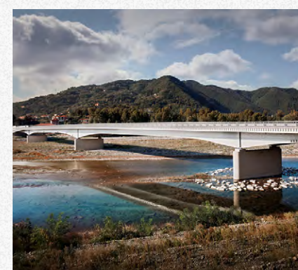
New Magra River Bridge Massa Carrara, Italy
